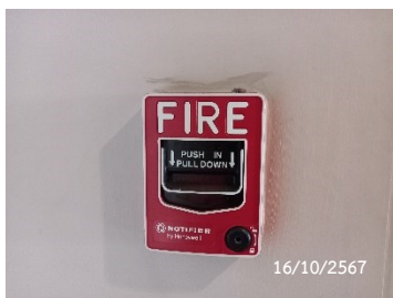
Fire Alarm Manual Station
