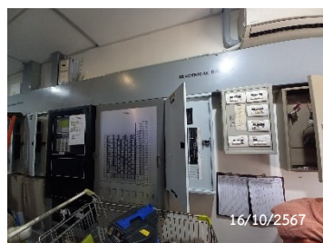
Graphic Annunciator Fire Alarm System
